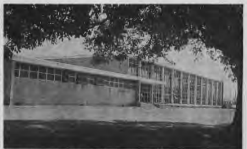
For future Southernites we built a foundation . . . .
