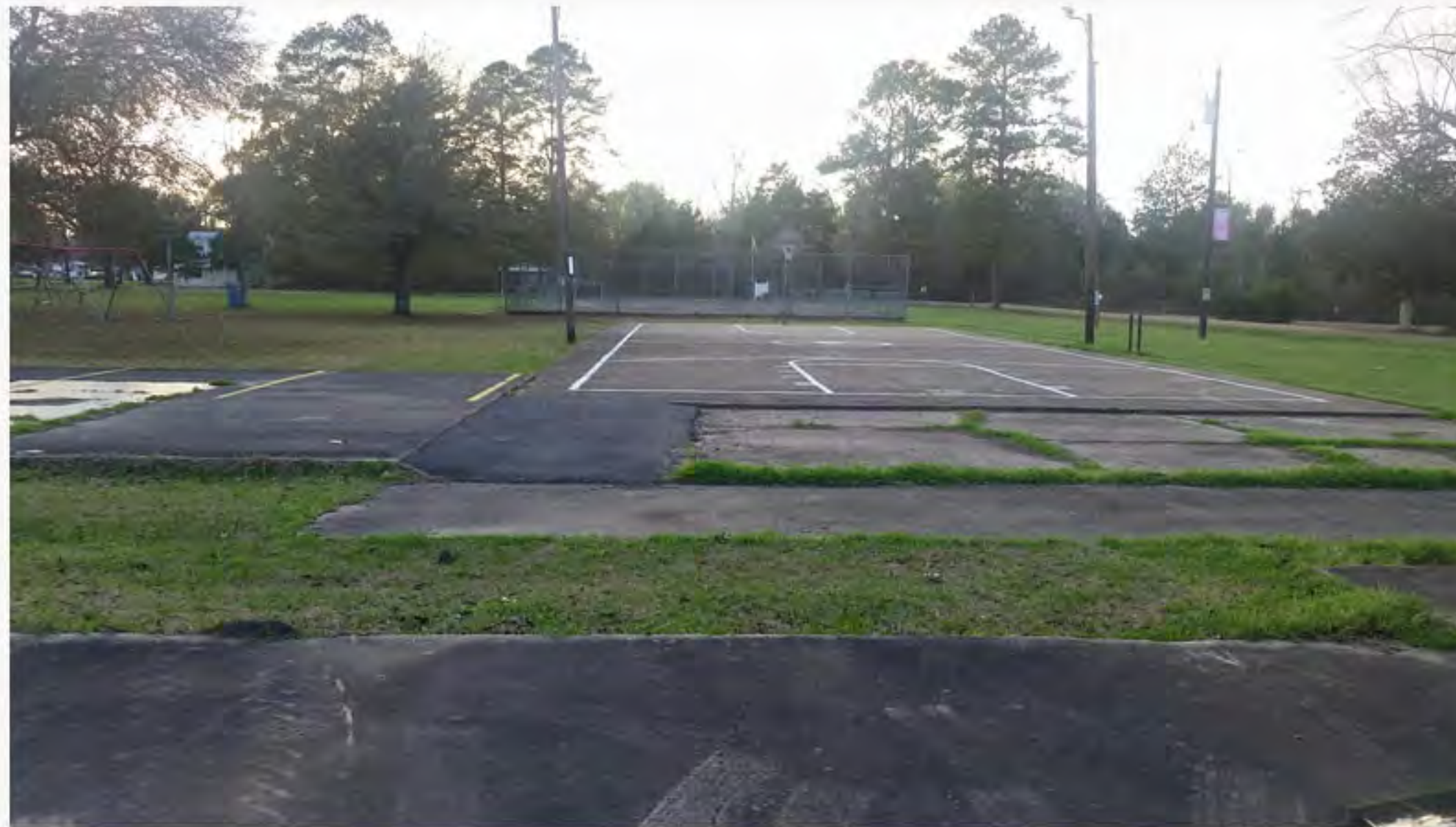
Foundation of the Former Charles P. Adams High School
