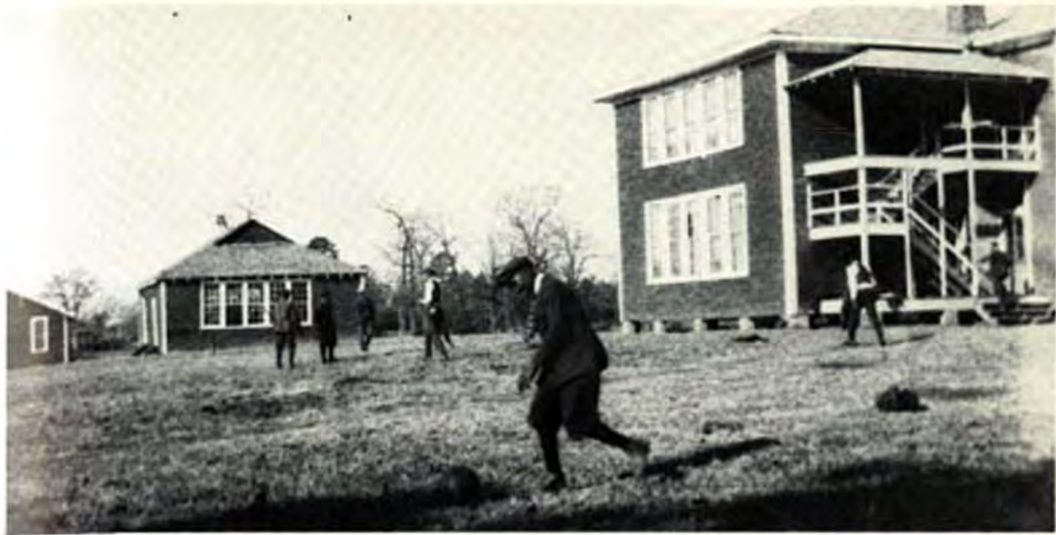
First School Building — 1916
